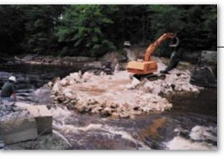
Over the next five weeks controlled blasting and removal of debris would take place, freeing up the river and exposing river features that would delight paddlers when the fall rains arrive.
